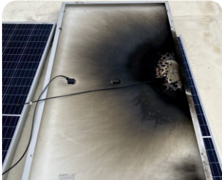
On-site Cutting And Welding
